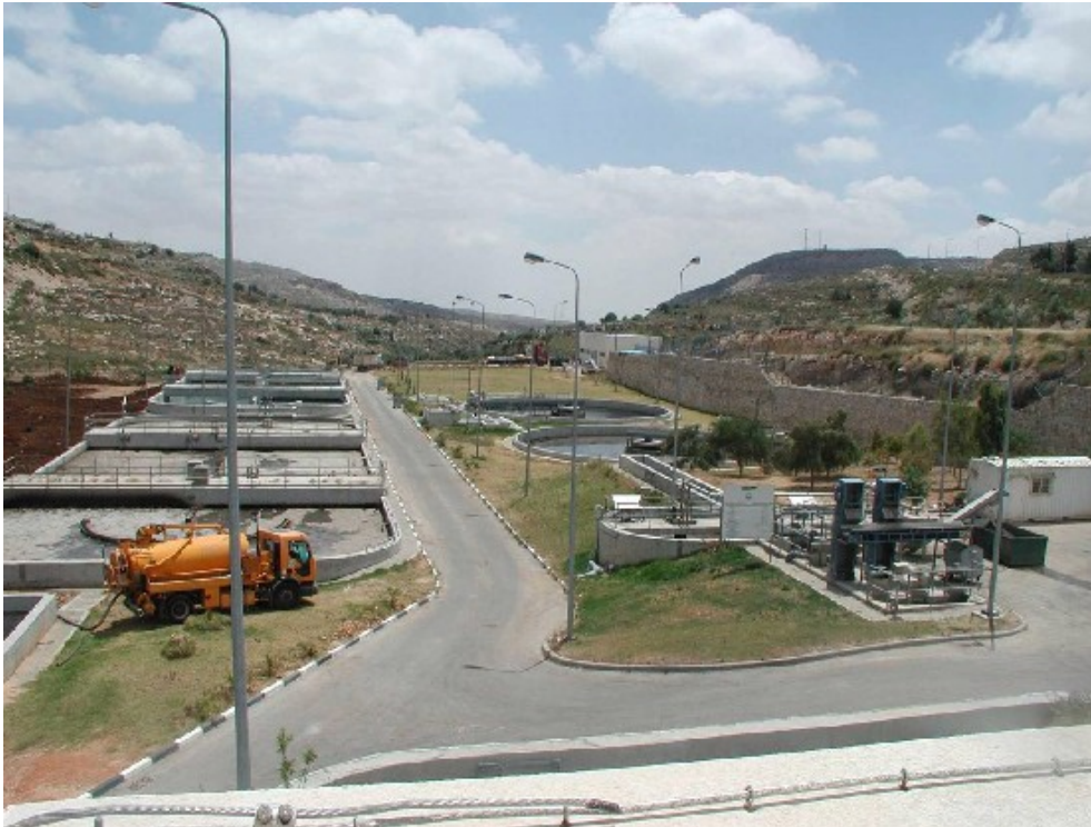
Photo 1.1 Overview of Al-Bireh WWTP
